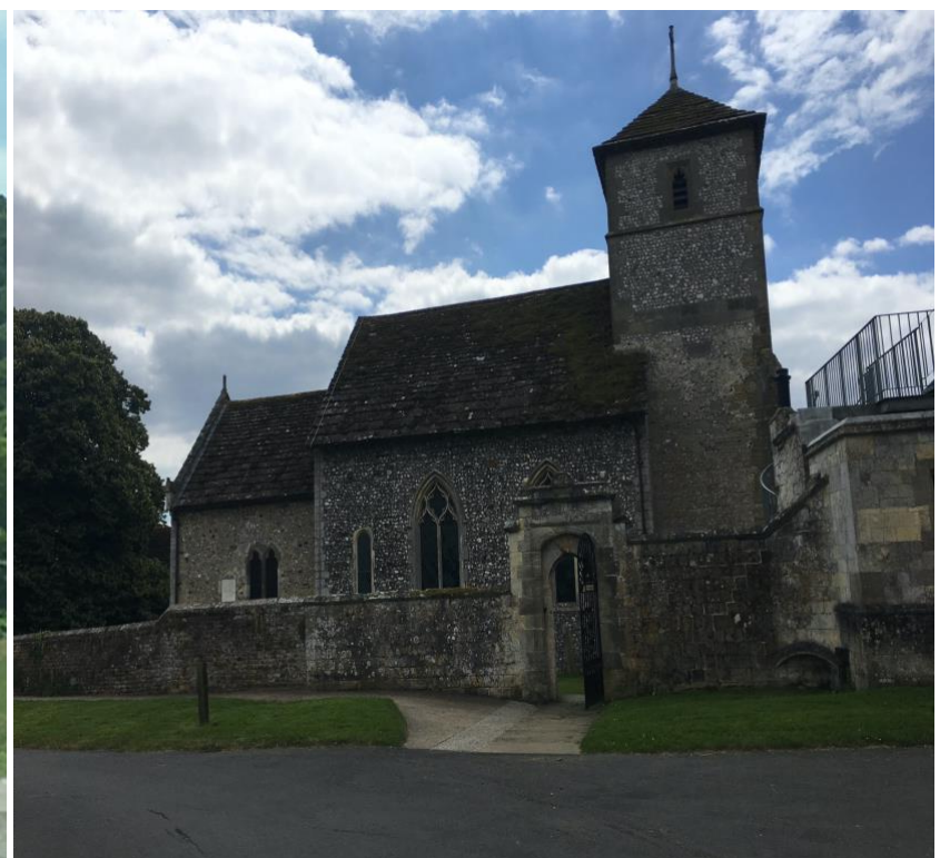
Above right: St Mary's Church
