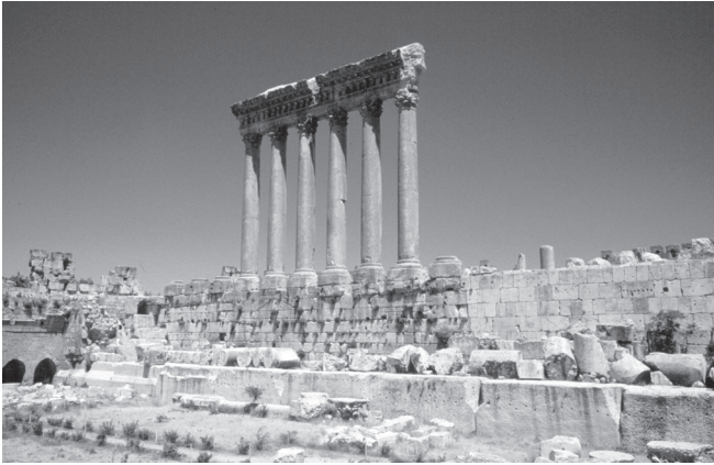
Figure 6.1. Heliopolis, Temple of Jupiter, south side, showing the six remaining columns of the peripteral colonnade of the temple in their original position at the edge of the earlier colossal podium. In front of this is a row of gigantic stone blocks that form the first course of the trilithon phase. Note that at the rear (left hand side in the photo) the dressing of the blocks has begun, but further along it has largely been abandoned, except at the junctions between blocks, where carefully-cut indentations provide a template for the dressing of these blocks. Photo by the author, 1994.
