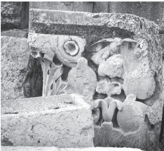
Figure 6.5. Unfinished anta from the temple of Jupiter. Note that the acanthus leaves on the left-hand corner are in a more completed state than the rest, and were perhaps more visible from ground level than the other features. Photo by the author, 1998.
