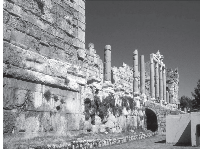
Figure 6.10. The propylaea of the Jupiter sanctuary. The original staircase has presumably been robbed out, exposing roughly-worked stones behind; the pilasters at top left have been left roughed out, ready for the final dressing of the surfaces.
