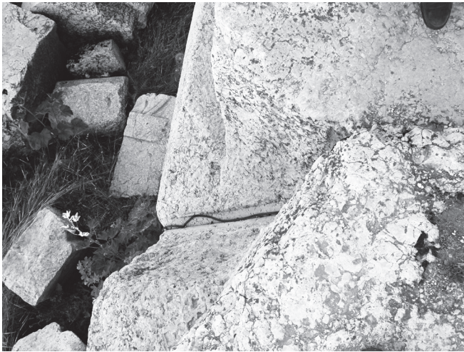
Figure 6.4. Another detail of the south side, showing the junction between two trilithon phase blocks and the indentation cut to serve as a template for dressing the lowest stage of the podium, viewed from above (and with a modern cable lying at the junction of the two blocks). Photo by the author, 2005.
