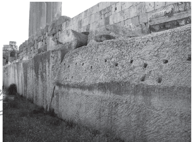
Figure 6.3. Detail of the trilithon blocks on the south side, towards the front of the podium. The nearest block exhibits the beginning of an attempt to dress it, whereas the others do not. Photo by the author, 2005.
