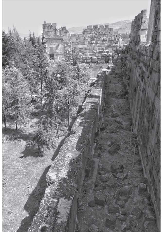
Figure 6.2. Temple of Jupiter, north side, showing the row of trilithon phase blocks and, on the right, the north side of the earlier podium, topped by the bases of the temple's columns built into the medieval fortifications. Photo by Niels Bargfeldt, 2011.
