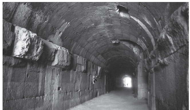
Figure 6.8. Vaulted passage beneath the great court. Photo by the author, 1995.
