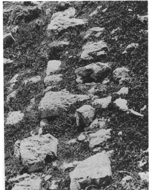
d. Building Wall
