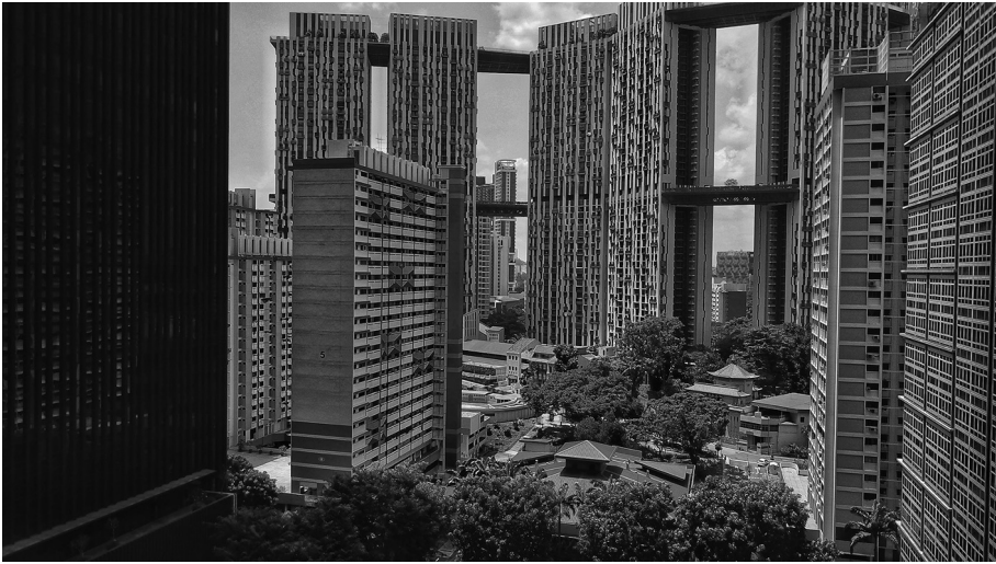
Figure 1.5 The Tanjong Pagar Housing Estate in Singapore is shown with the Pinnacle@Duxton in the background.
