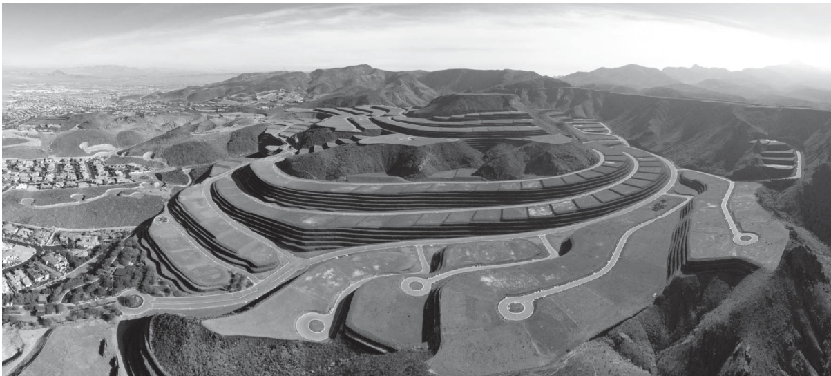
Aerial image, taken in 2015, of the incomplete Ascaya development in metropolitan Las Vegas.
