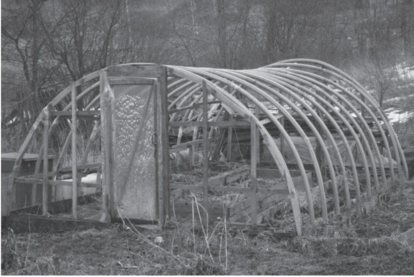
FIGURE 0.2. Walk-in greenhouse frame, made of fiber-optic cable casing. Image courtesy Elena Tipikina.
