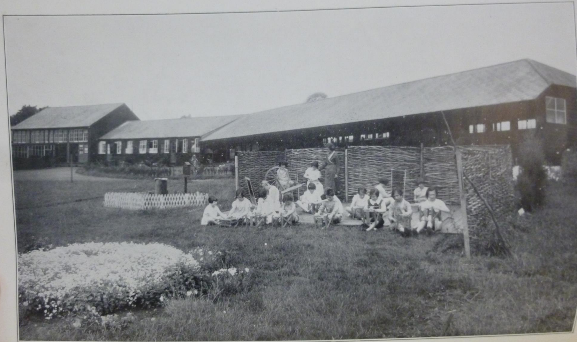
A SECTION OF CORLEY OPEN-AIR SCHOOL.
