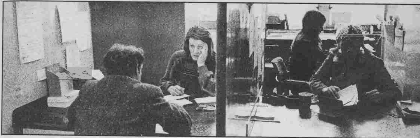
Keyworth House labour exchange
