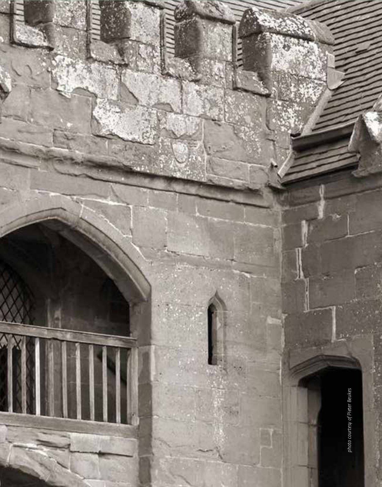
The Gatehouse Balcony at Stoneleigh Abbey
