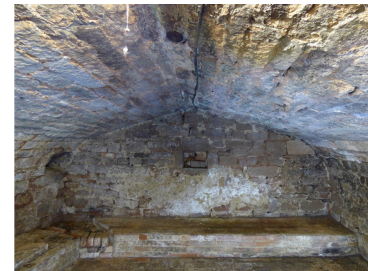
Fig. 5. The cellar N wall, note the blocked openings in the centre of the wall and to the left.
