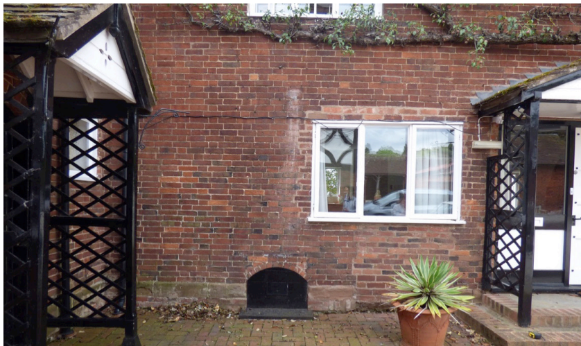
Fig. 3. The SE end of the N range, showing the site of an earlier door, behind the flowerpot, and the coal-shoot for the cellar.
