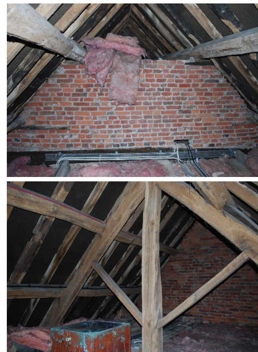
Fig. A4. The early nineteenth century roof structure, showing reused smoke-blackened rafters (photos James Edgar) (a) looking north (with brick partition wall); (b) Rafters beside king post.
