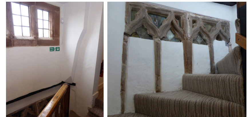
Fig. 12. The staircase, showing the cut-back wall and upper window, left, and pair of blocked windows with glass still in place, right.
