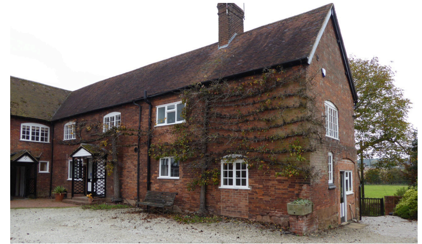
Fig. 1. The N range of Cryfield Grange, from the NE.
