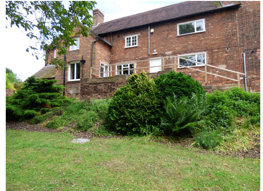
Fig. 8. The W side of the N range, showing the inserted doorway and concrete steps.
