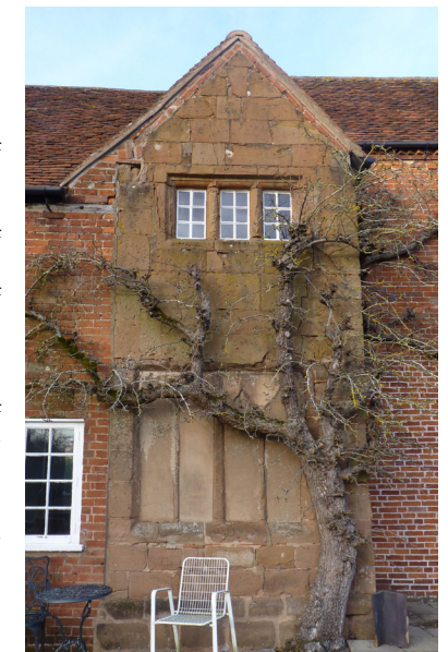
Illustration 10: Tracery window head at Cryfield Grange Photographed on 22/2/2017 by N. W. Alcock
