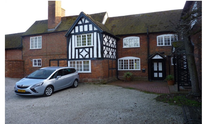
Fig. A1. North view of Cryfield Grange (2017)
