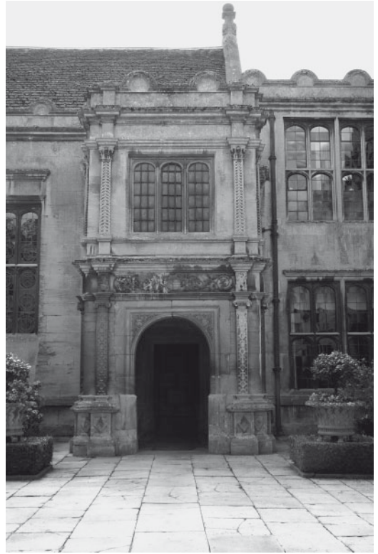
12. Deene Park, porch from the courtyard.
