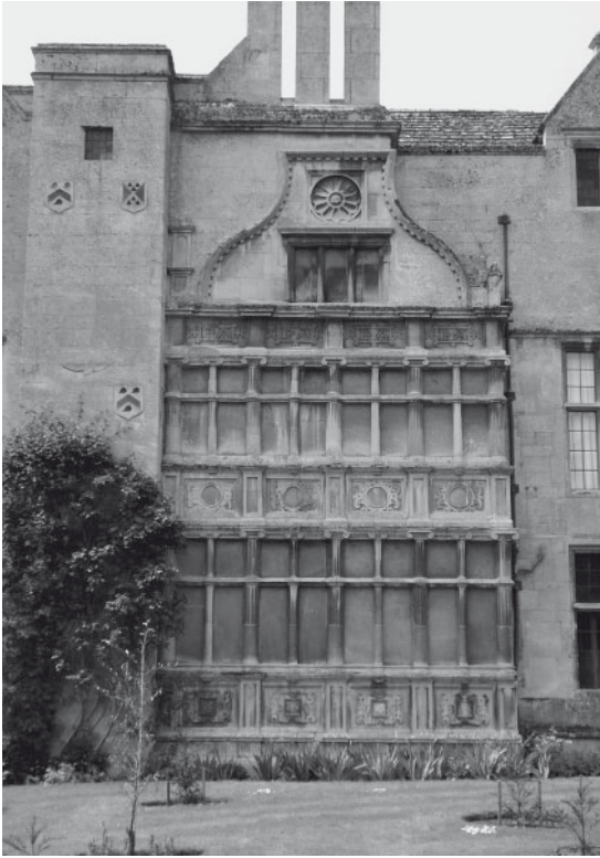
11. Deene Park (Northamptonshire), bay window with glazing infilled, now sited on the east front.
