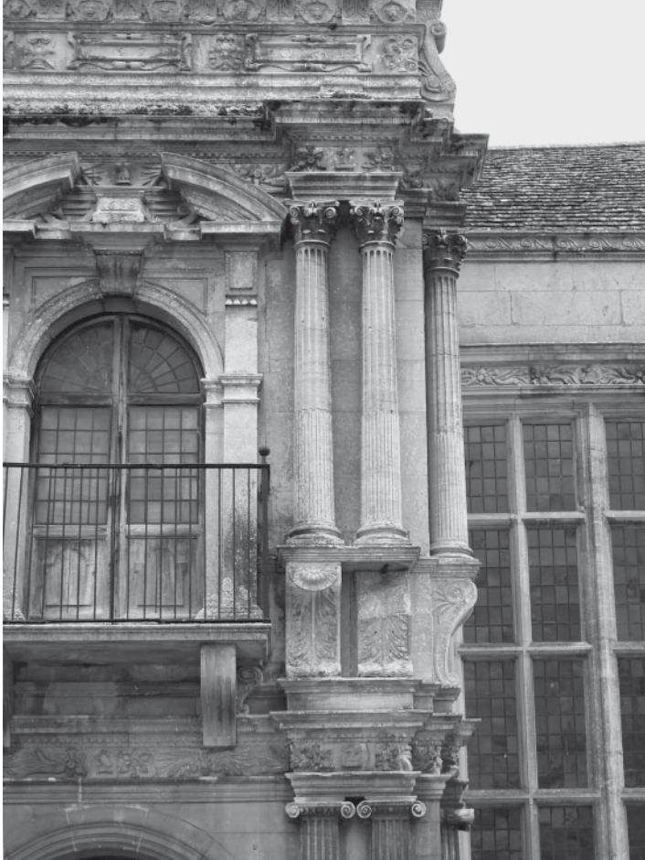
19. Upper level of the hall porch, Kirby Hall.
