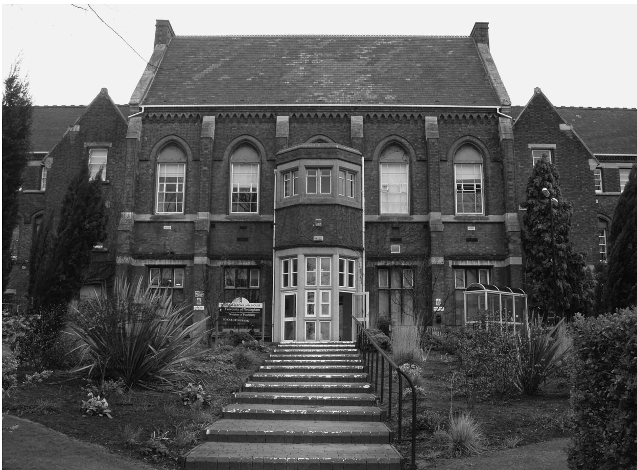
PLATE 2: Mapperley Hospital chapel and hall of the 1880 wing from the south west.
