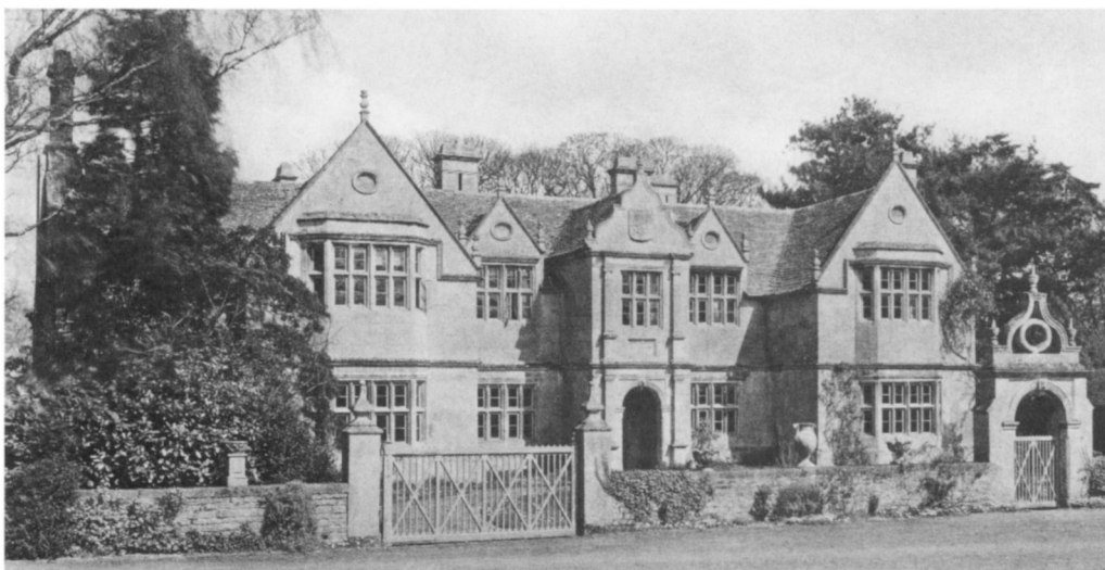
Fig. 16. Stibbington Hall, general view (Photograph 1914)
