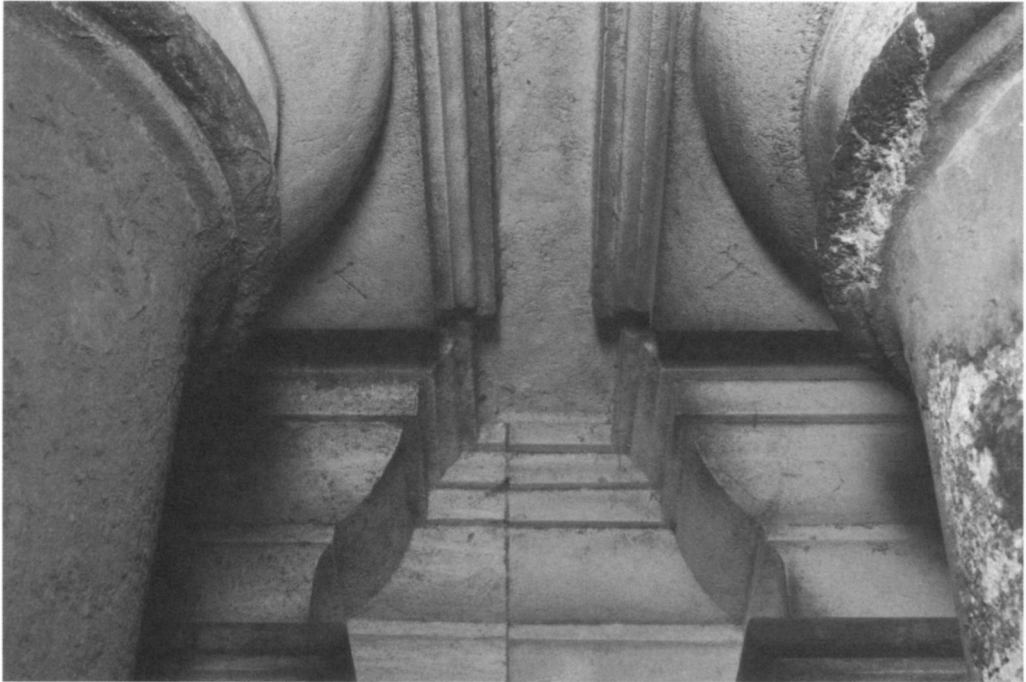
Fig. 7. Apethorpe Hall, mark 2t7 on the undersides of impost blocks, east range, west porch (Photograph 2006, by Patricia Payne)
