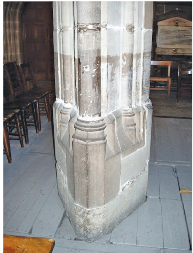
PLATE 7: Nottingham St Mary, nave pier base.
