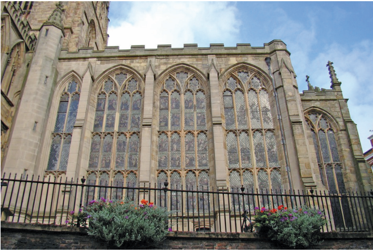
PLATE 5: Chancel exterior from the south showing the medieval windows reset in the early 20th-century aisle.
