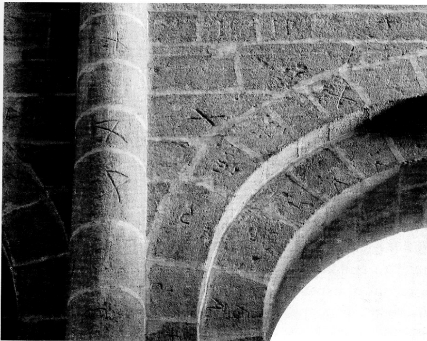
2.1. Masons' marks on the vaulting shaft, arch and spandrel wall of the transept arcade in the cathedral of Santiago de Compostela, Spain [Author].
