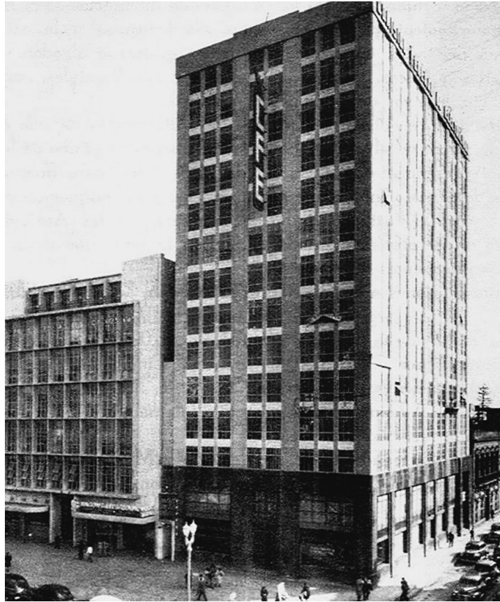
FIGURE 4.2. CFE administrative center, 1960
