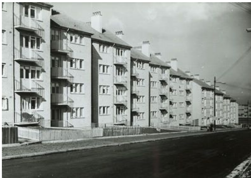
Image 6: Corporation Housing at Birgidale Road, Castlemilk, 1958 (Glasgow City Archives: a)
