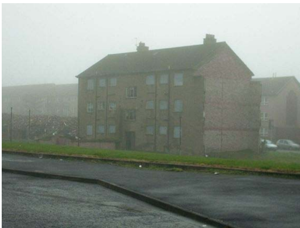
Image 9: Demolition work on Inverlochy Street, Garthamlock, September 2006 (Paice, 2006)
