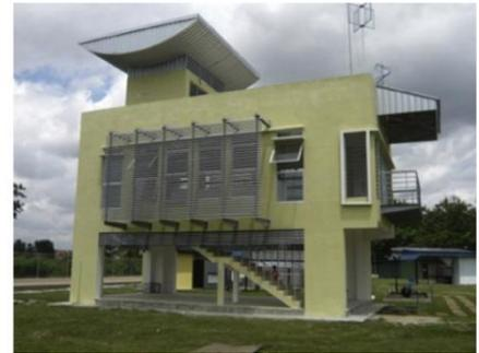
With advanced natural ventilation design, high air change rates can indeed be achieved, even with low incident wind speeds (see example with CFD modelling from Malaysia).
