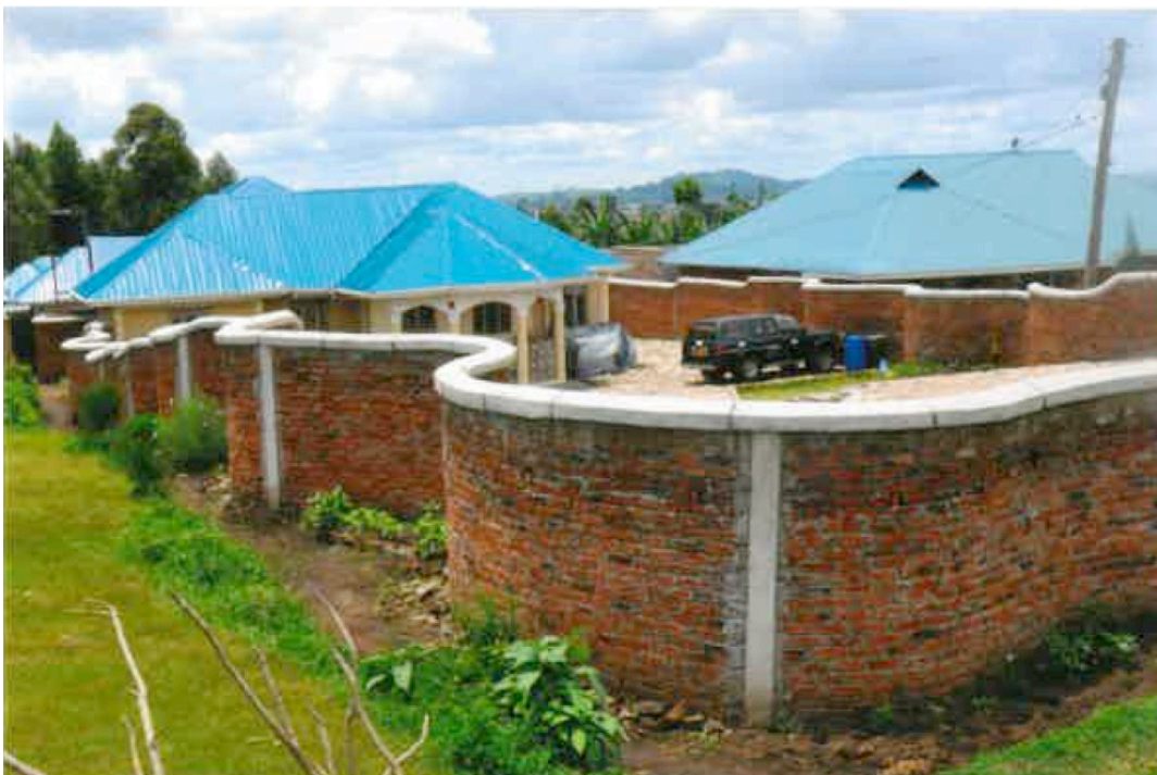
Fig 3 Serpentine boundary wall in seismic zone (Fort Portal, Uganda 2015) 100mm-thick
