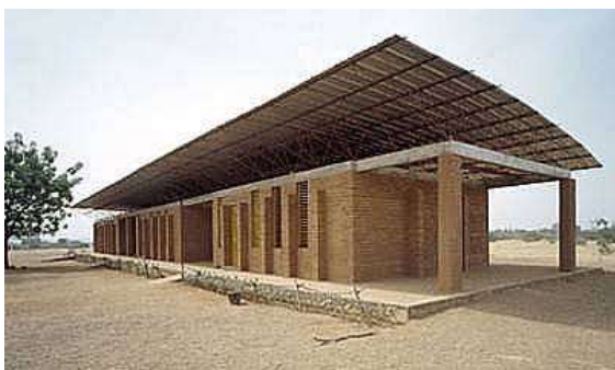
Grando School, Burkina Faso: earth blocks, passive cooling, source: Patti Stouter
