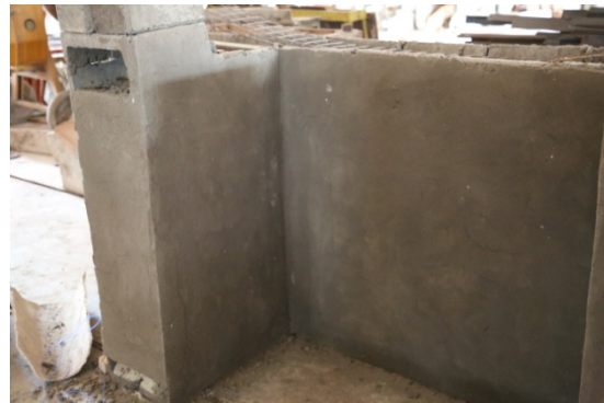
A demonstration wall of compressed mud interlocking bricks built at NHBRA - Tanzania plastered in mud mortar ready for further finishing coats.
