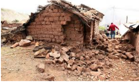
Houses damaged by ground shaking
