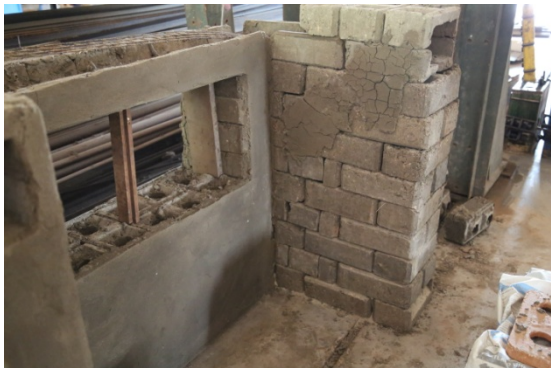
A demonstration wall of compressed mud interlocking bricks built at NHBRA - Tanzania plastered in mud mortar ready for further finishing coats.
