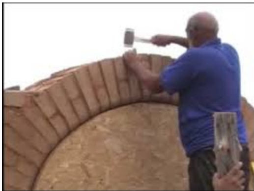
Bridging the openings with arches
