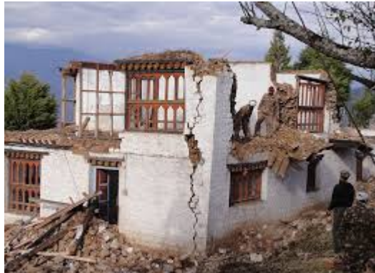
Mud brick houses are easily destroyed by natural disasters
