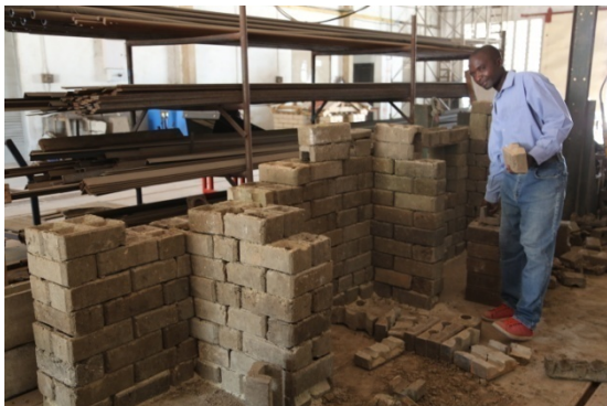
A demonstration wall of compressed mud interlocking bricks built at NHBRA - Tanzania
