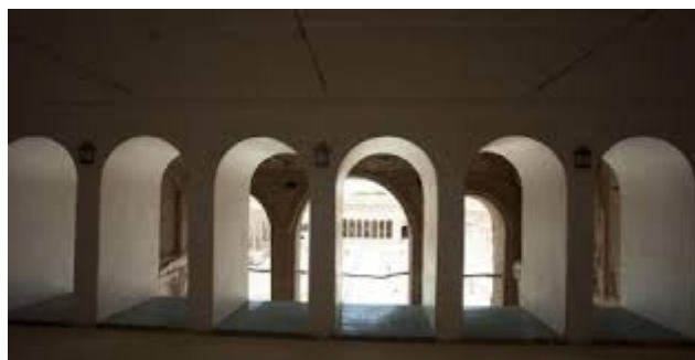
Bridging the openings with arches
