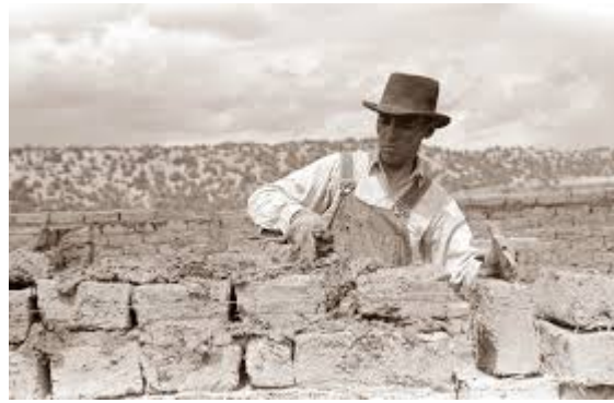
Construction process for mud brick house
