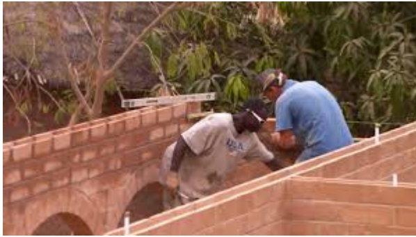
Multiple and large openings can be bridged by arches and beams
