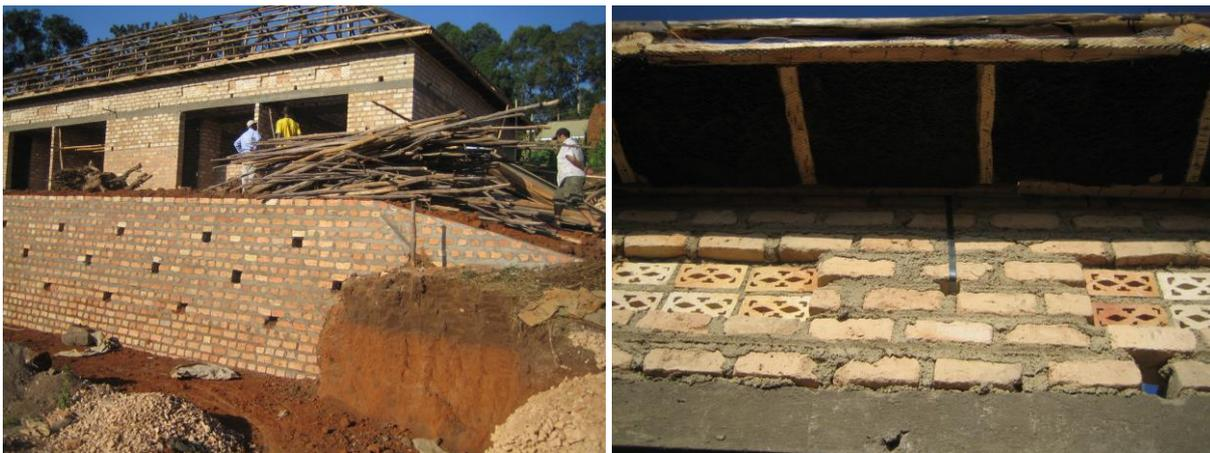
Figure 5: Mortar thicknesses of up to 30mm is normal for brick walling (Uganda)
