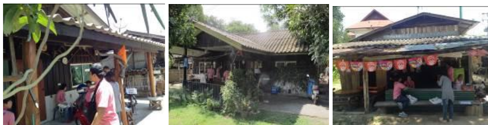
Fig. 2 single story wooden typical houses in the northern region
