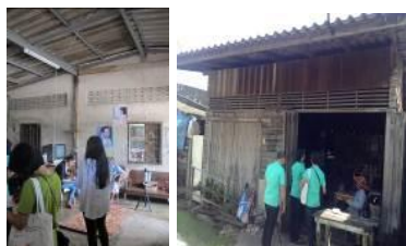
Fig. 8 Roof and ceiling of houses in the southern region
