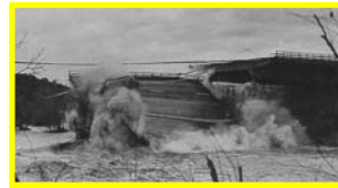
Schoharie Bridge, USA 1987
