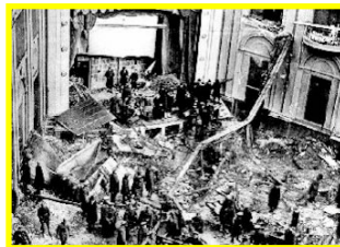
Knickerbocker theatre roof collapse, 1922
