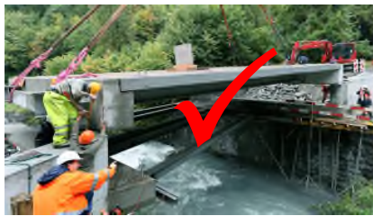
Avançon Bridge (Bex, Switzerland), GFRP face sheets and balsa wood core
