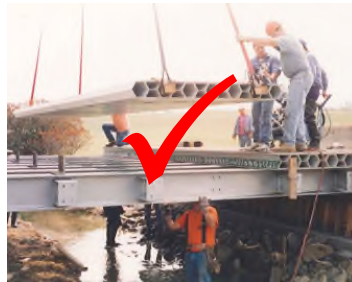
Sandwich panels (web- or homogeneous-core)
