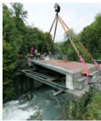
Avançon Bridge (Bex, Switzerland), GFRP face sheets and balsa wood core
