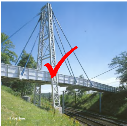
Kolding Bridge, Denmark
