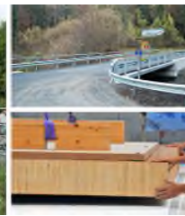
Avançon Bridge (Bex, Switzerland), GFRP face sheets and balsa wood core
