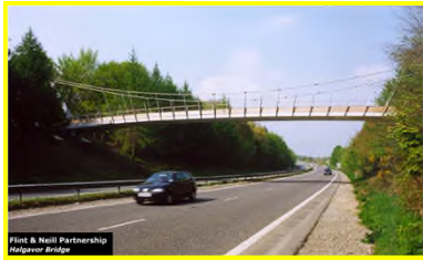
Frost & Neill Partnership Halgavor Bridge
