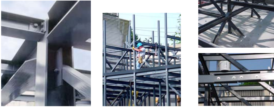
Figure 1. Frame connections for structures of pultruded shapes ([4] and [5]).
