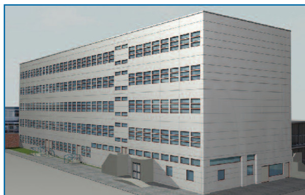
Over-clad building using 'rain screen' metallic cladding.
