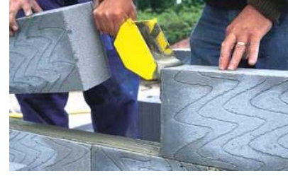
C – Thin mortar joints
