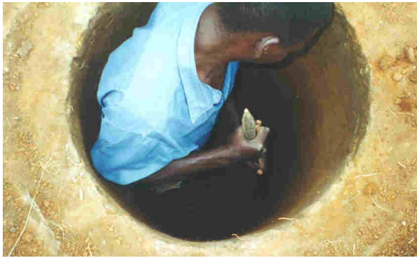
Figure 1 Excavating the tank
