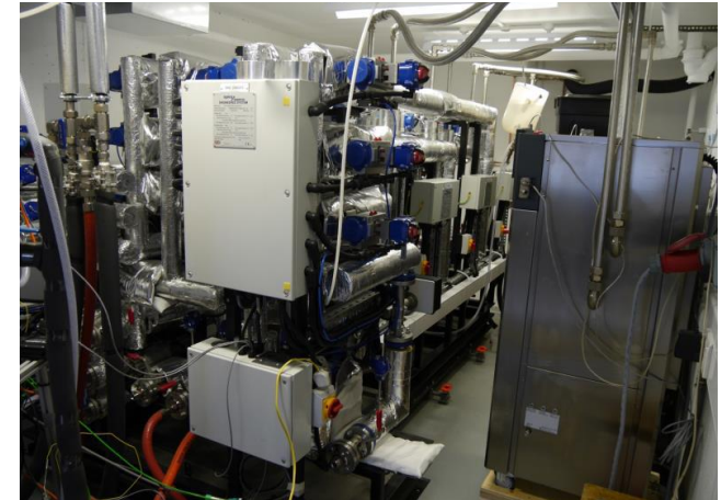
Heat exchanger tests
