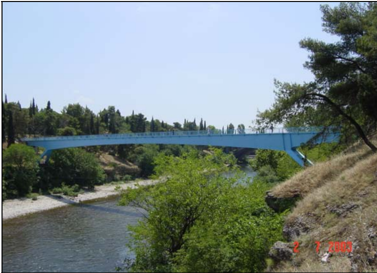
Figure 1: Photograph of the Podgorica footbridge.
