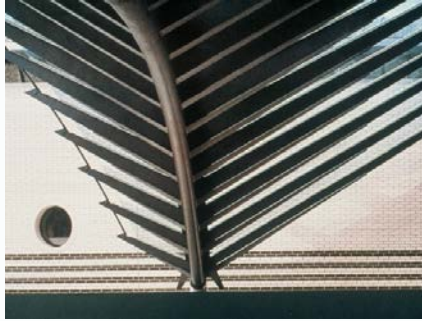
Canopy entrance to School in Wohlen, Switzerland. Design: Calatrava, 1980
