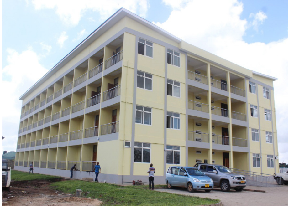
The newly constructed student hostel building at one of the universities in Tanzania, built in response to recommendations based on the outcome of a TCU quality audit of the university.
