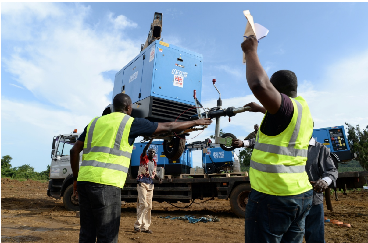
Constructing a UK treatment centre in Sierra Leone
