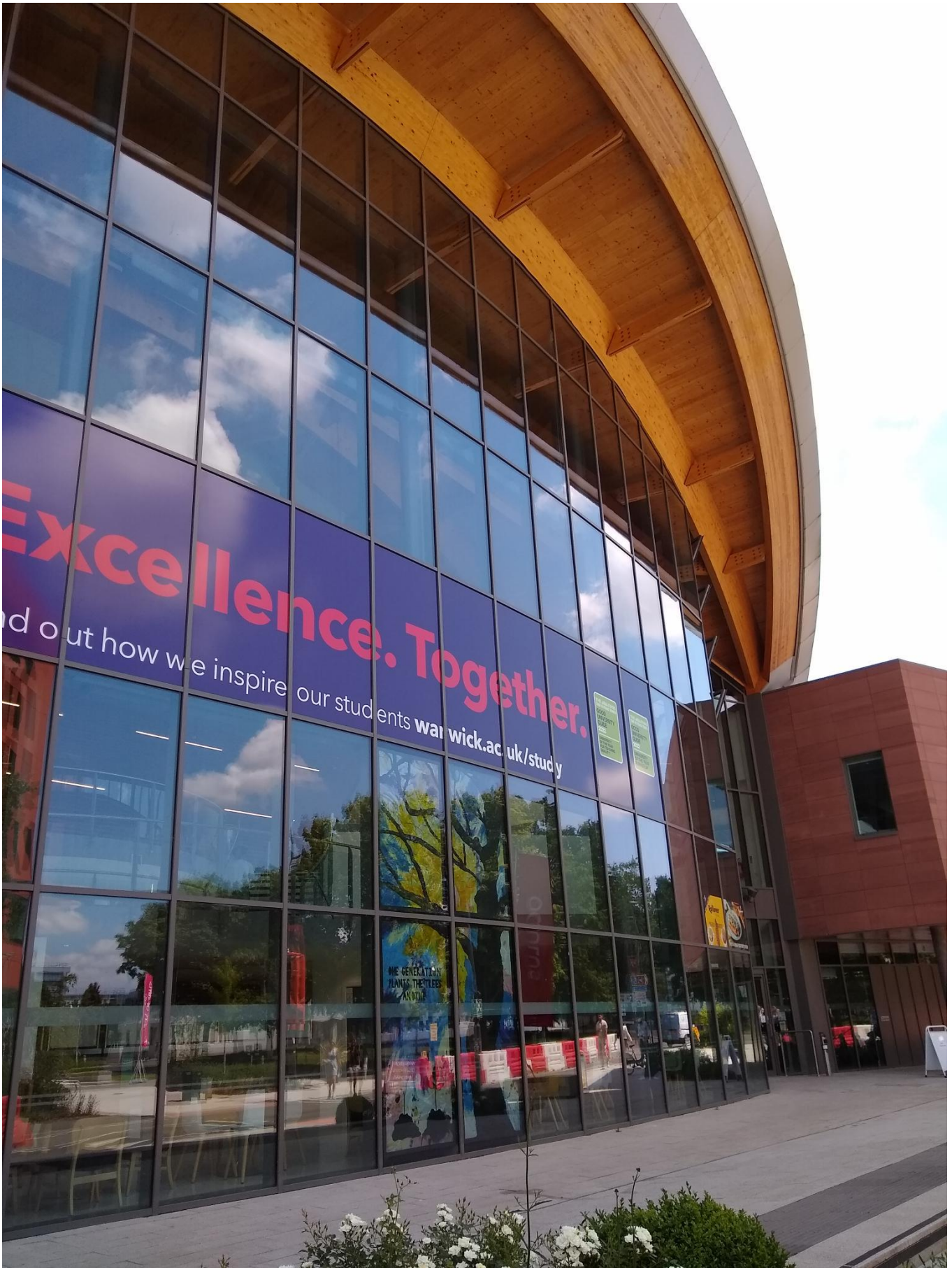
Oculus Building, main campus
