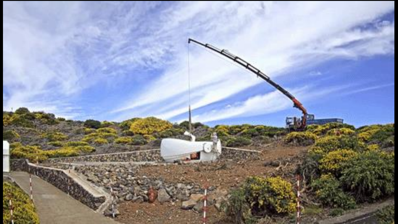
Installing GOTO on La Palma Credit: Paul Chote
