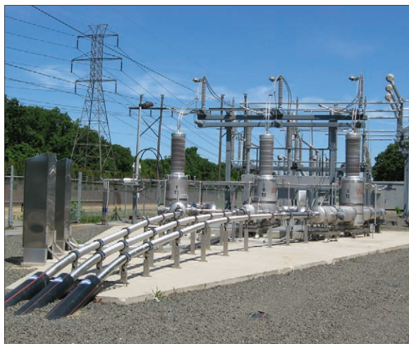
Laying the ground work The Holbrook Superconductor project at a substation in Long Island, New York, has been operating with some 160 km of superconducting cables since 2008.
