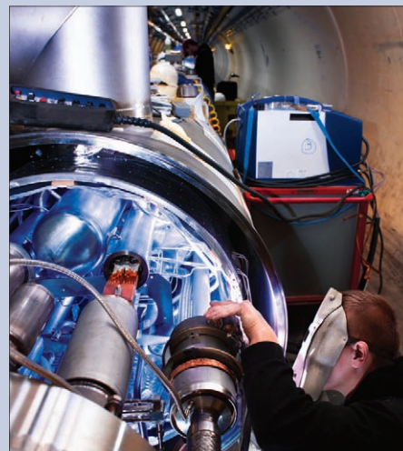
Interconnected A welder works on the junction between two of the Large Hadron Collider's superconducting-magnet systems.
