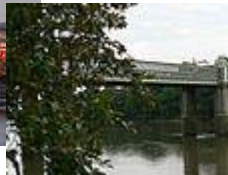
Kew Railway Bridge, 1869
