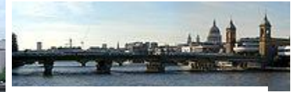
Cannon Street Railway Bridge, 1866
