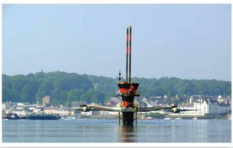
Tidal turbine, Strangford Lough, Northern Ireland, generating electricity from tidal streams was plugged into UK's national grid in July, 2009
