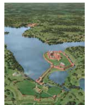
What Kenilworth Castle with the mere restored might look like.
