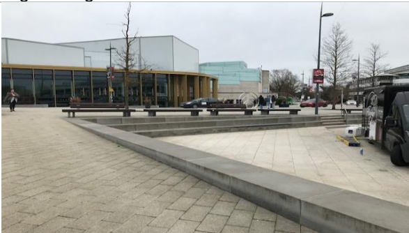
Large steps around two thirds of the site.
