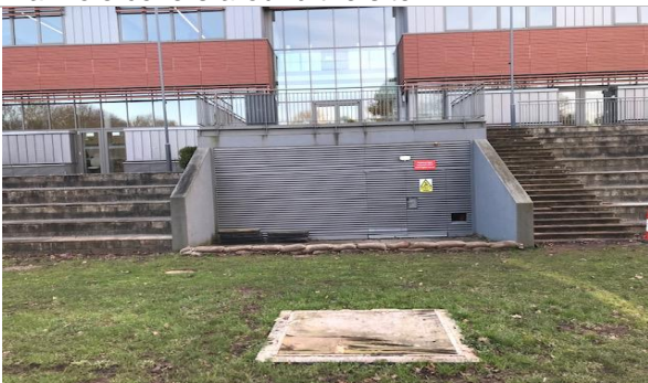
Plant room with raised concrete platform to the entrance
