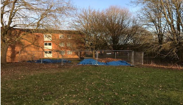
Fenced off area in the North Corner
