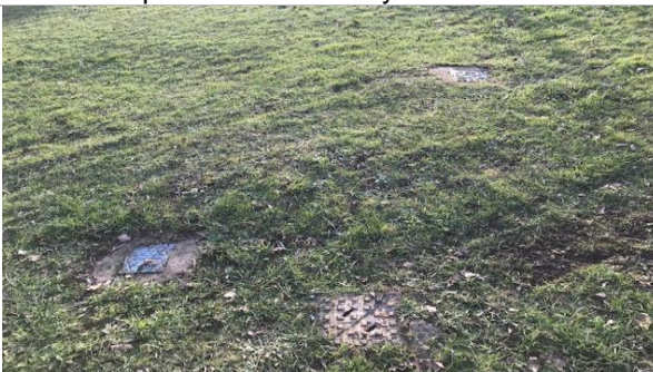
Manhole covers around the site.
