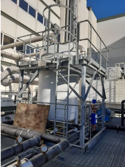
External lower roof area with fixed ladders
