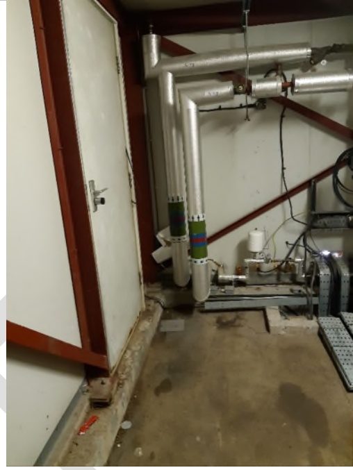
Roof access door at top of stairs
