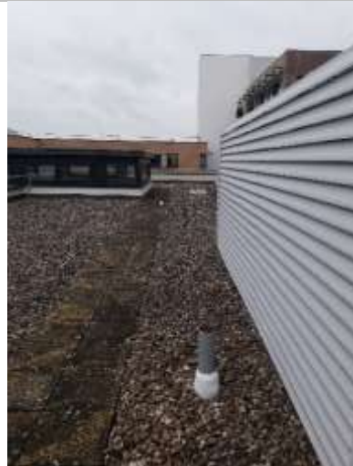
Walkways and vents protrusion
