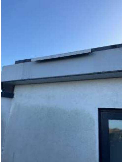
Potential ladder access platform onto secondary roof.
