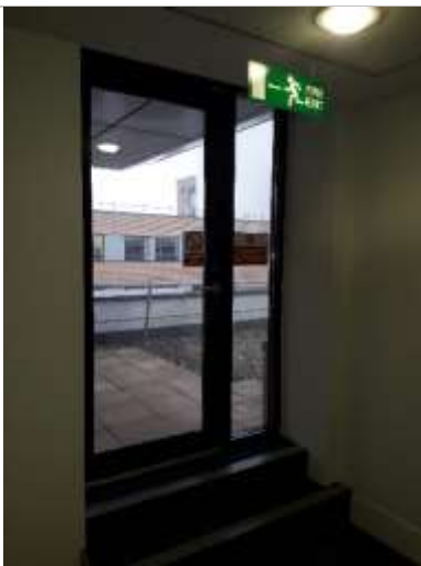
Internal view of roof access
