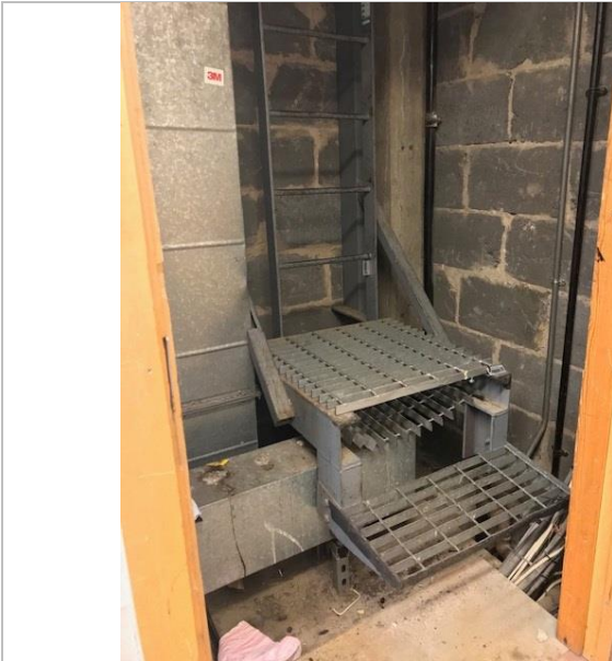
Steps leading to Galvanised Steel fixed ladder
