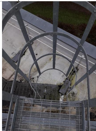
Galvanised Steel fixed ladder leading to the higher roof.
