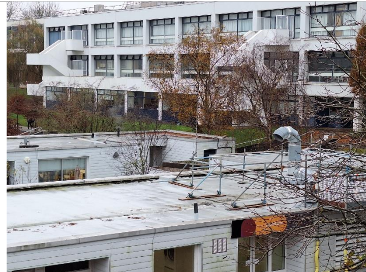
Roof with flue
