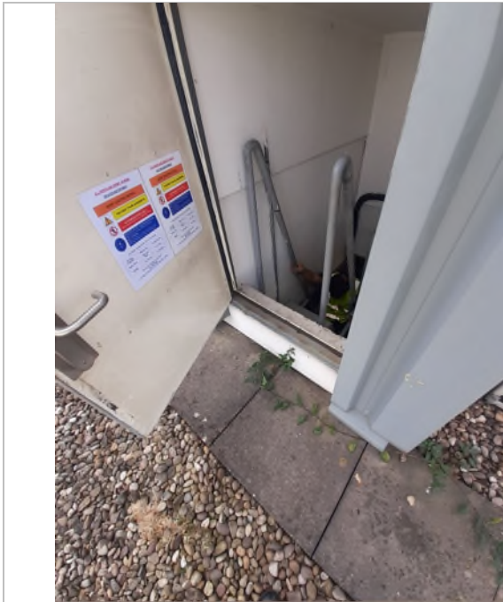
Roof access door and steps
