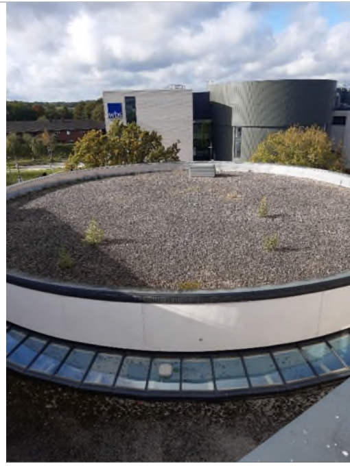
Lecture theatre roof (viewed from main roof)
