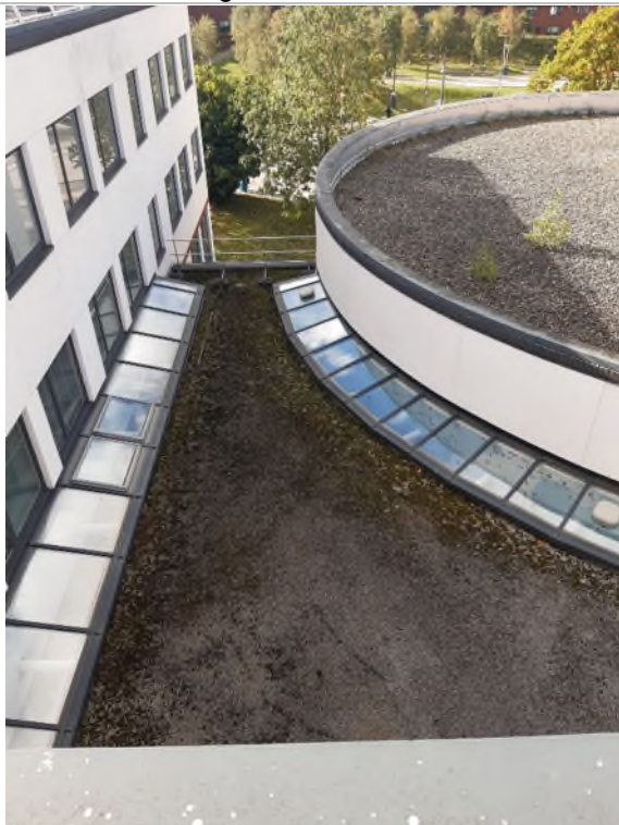
View from main roof to atrium and lecture theatre roofs
