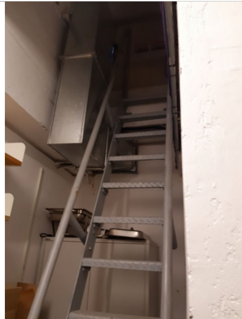
Fixed steps in 3.27 to roof door
