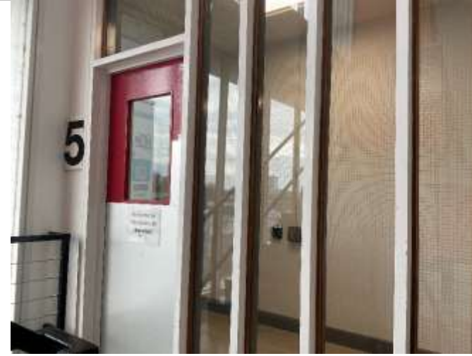
5 th floor entrance from stairwell
