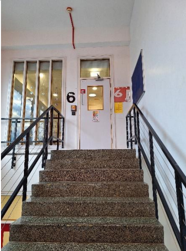
6 th floor kitchenette entrance
