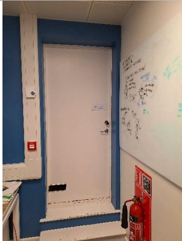
Roof access door with Salto in B600
