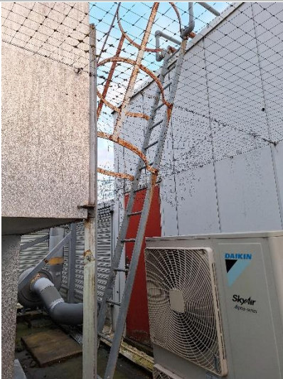
Access ladders leading to Science Block B roof
